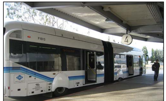
Figure 3. The El Monte Bus Station
