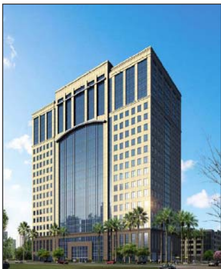
The Platinum Tower, approved in October 2007, is a 20-story office building encompassing nearly 600,000 square feet.
