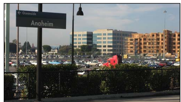
View from the Metrolink station across the Angel Stadium parking lot. Projects such as the one under construction 2100 at Platinum Triangle will surround this city-owned surface lot with transit-oriented development.
