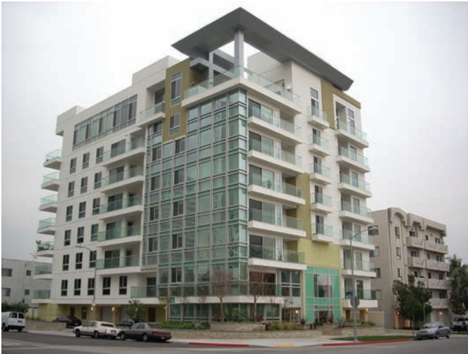
This Koreatown residential high-rise in Los Angeles illustrates why Los Angeles enjoys higher intensity land uses when compared with Portland's outlying station areas
